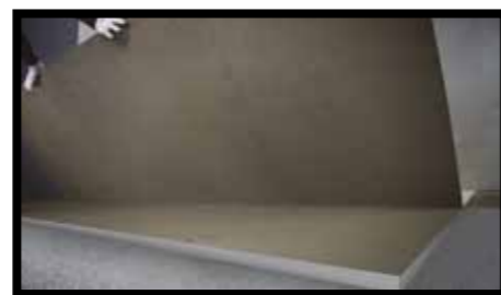
Fig.32 - Rest the slab on its long side and guide it down towards the floor.
