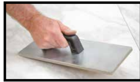
Fig.30 - After laying the tile, make sure it is firmly bound to the underlying surface to prevent gaps and air bubbles forming. For this purpose you must use a tile beater with a rubber bottom (for example Raimondi "142G").
