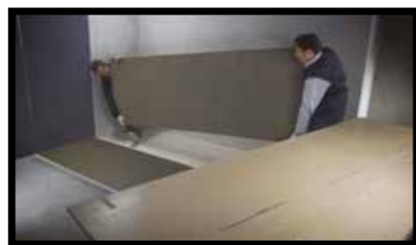
Fig.31 - To handle tiles, raise them to their upright position, whilst grasping them from the top edge. They can then be moved with the help of a second person.
